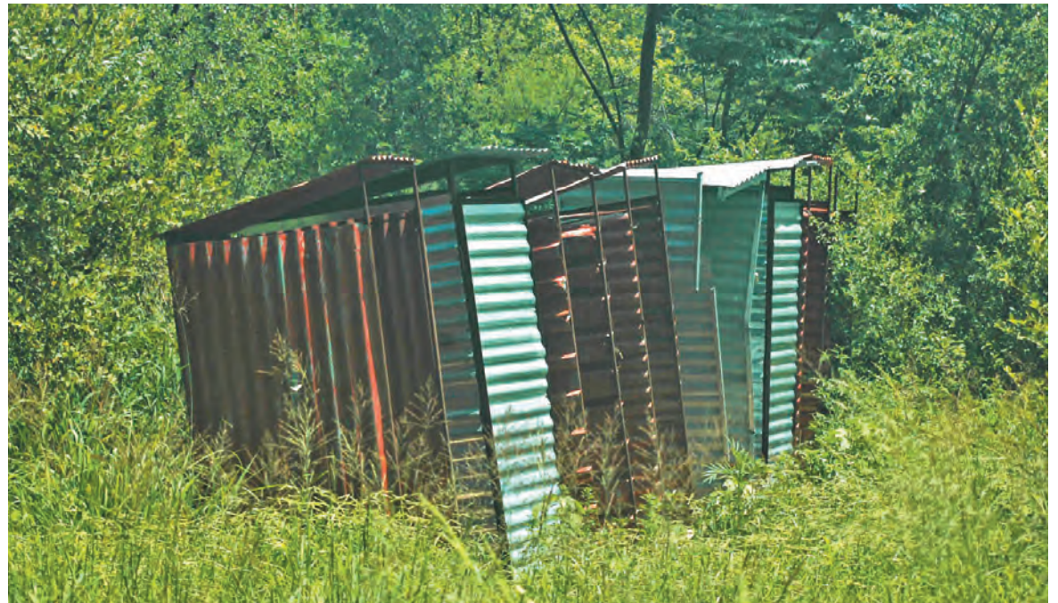
The dilapidated structure – located in thick grass – that the pupils from Reahlahlwa Primary School used for many years to relieve themselves.
