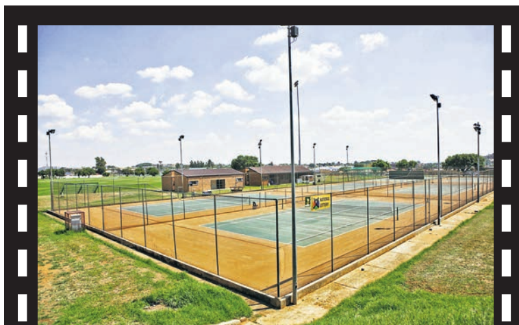
The commission made it possible for the construction of this multi-purpose court that caters for tennis, netball, volleyball, a gymnasium and athletics tracks
