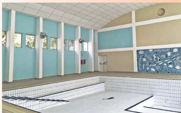
The centre at Bunting Road was built at a cost of R7-million, of which the NLC contributed half.
